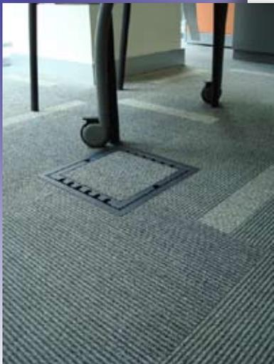
The RBC/RBTT project in downtown Port of Spain, Trinidad is an example of new generation building design. Utilizing a fully modular foundation backbone to include ASM access floor, PowerLink, and DataLink systems has and will enable the end user to expand, redesign, and adjust as needed in a fast paced environment.
